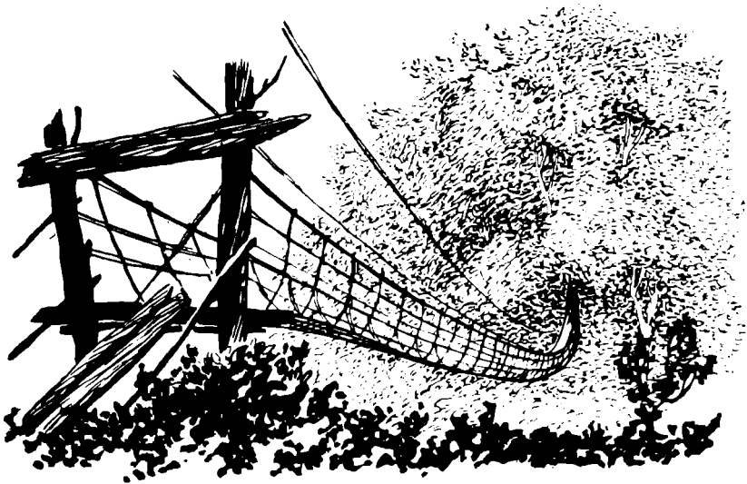
A cane suspension bridge in the Dibang Valley
